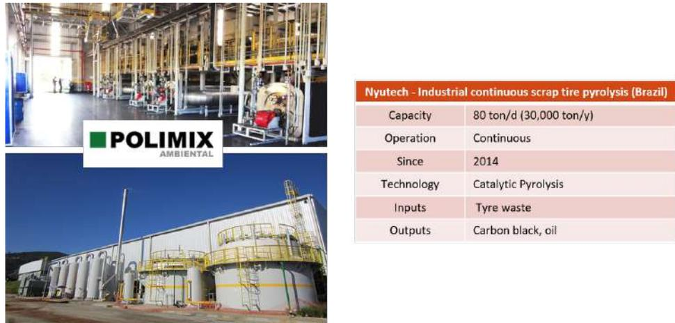
Figure 61: Description of industrial continuous scrap tire pyrolysis plant in Brazil.
